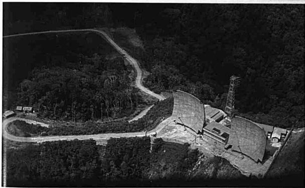
Top, a rural access road which opens up the interior while at the same time provides the farmers with a faster means of transporting their produce to the market, and bottom, a tropo-scatter station which receives TV signals for onward transmission, through the micro-wave system, to other parts of the State.
